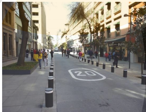
Fig.24: Avenue 16 de Septiembre - Mexico City, Mexico, Photo courtesy of Institute for Transportation and Development Policy - Streets as Places Strategies: Narrow vehicle lanes • Low vehicle speeds • Buffers between pedestrians and vehicular traffic
